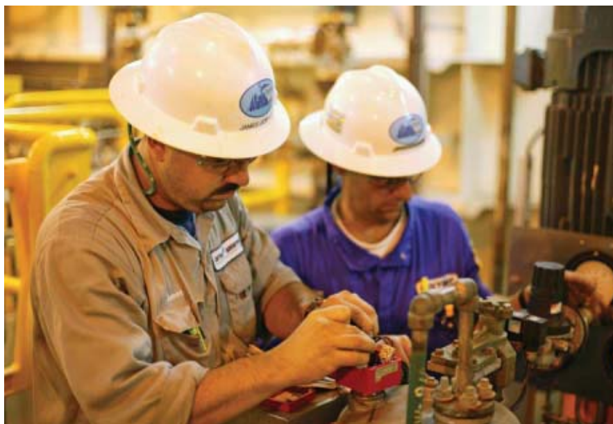
Maintenance work at Atlantis
