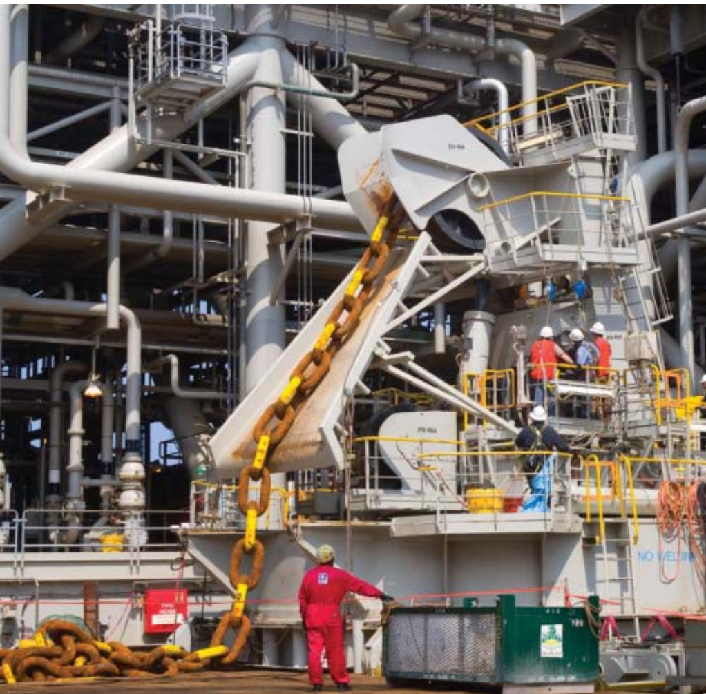
Technicians Service the Steel Catenary Risers Pull In Unit at Atlantis
