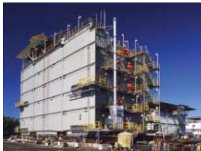
Construction of living quarters
