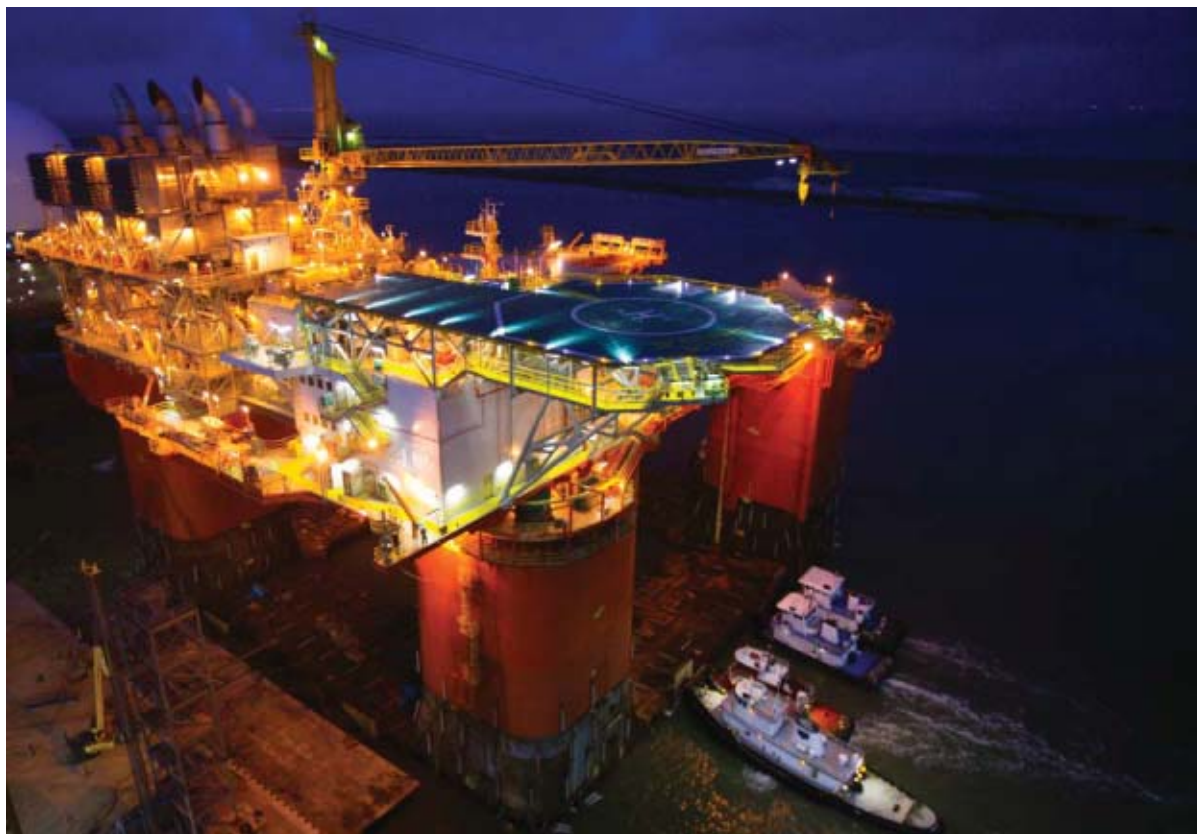
Platform final assembly in Ingleside TX
