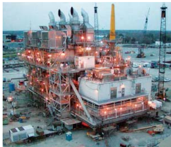
Fabrication in Morgan City, Louisiana.
