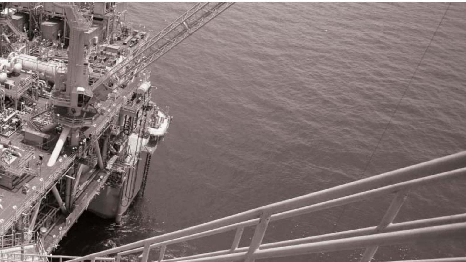
Cover - Atlantis Production Quarters Platform, view from the flaring tower.
