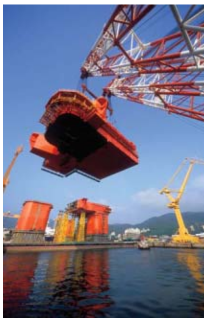
Atlantis hull during assembly at the DSME yard in Korea.
