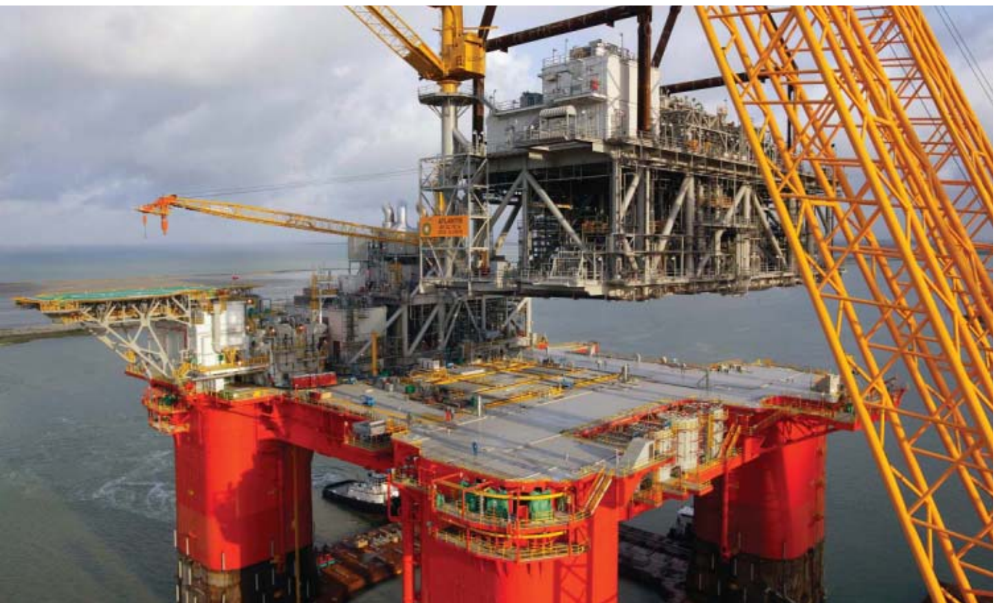
Ingleside, TX. Installing the gas compression unit on the platform.
