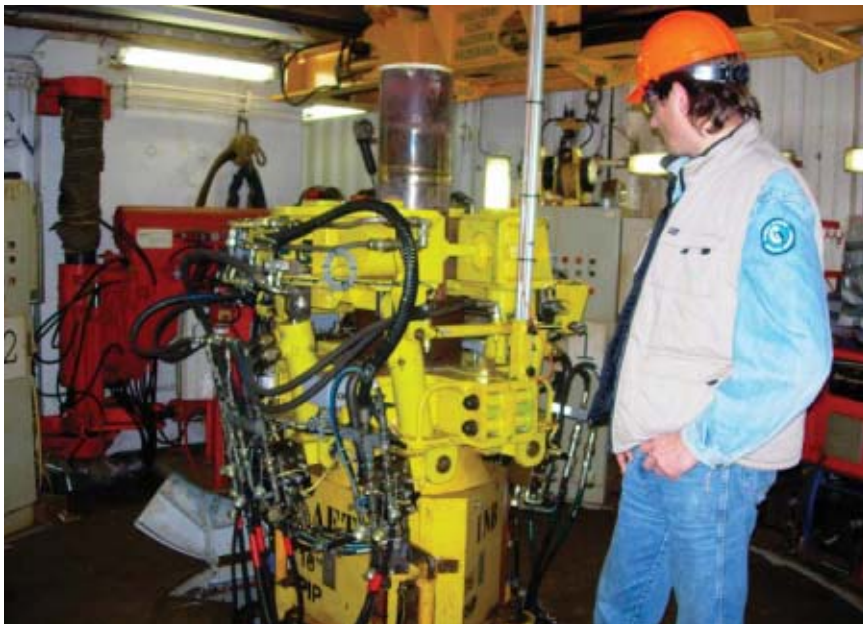
Inner pipe fixation tool 'OBELIX' installed in welding station
