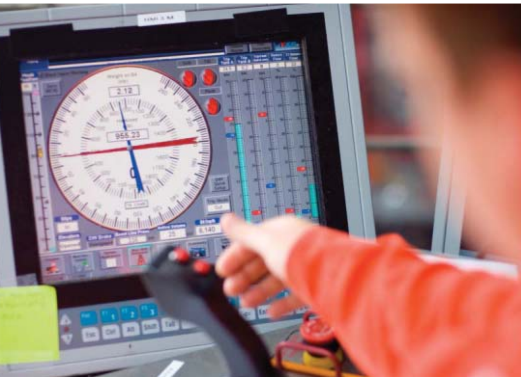
The Cyber Rig Drillers Console on the Transocean's GSF Development Driller II.
