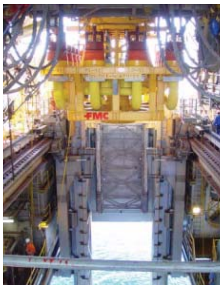
A "compact" manifold design allowed efficient installation from the drilling rig.
