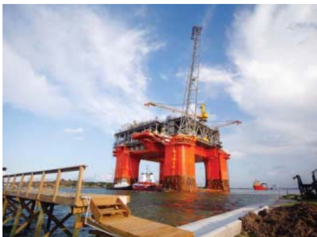
Installation of the generation unit at Ingleside TX.
