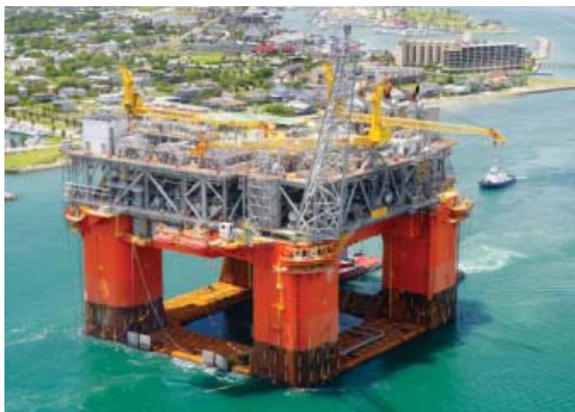
Atlantis, with Mustang-designed topsides production facilities, begins its journey into Gulf of Mexico waters.
