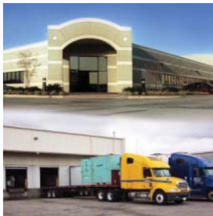
Top: Office & training center in Harahan, Louisiana. Bottom: Delta Catering operates a state-of-the-art warehousing & distribution center.
