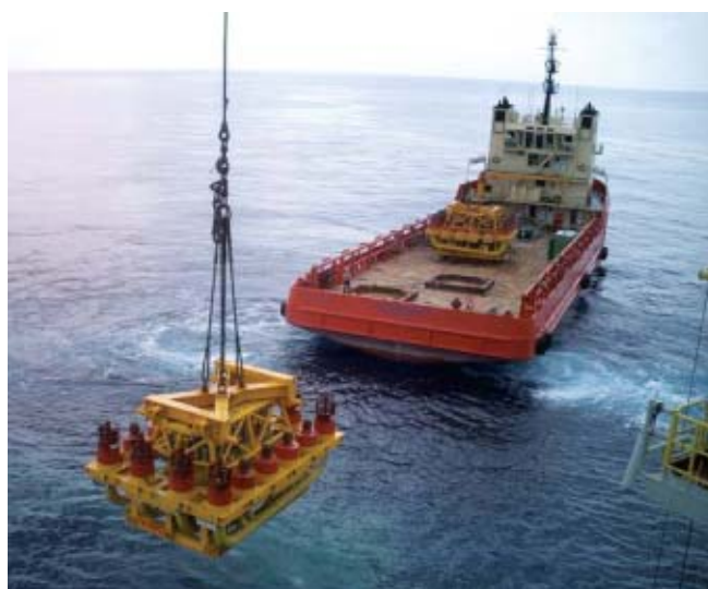
DDII performing subsea component installation
